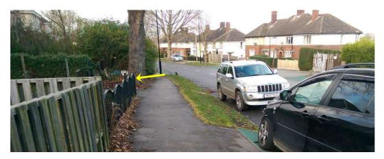
It will not be possible to construct the paved strip as indicated due to the severe gradient. In order to provide passenger access between the footway and bus-stop, significant civils works will be required. There will be a need for the provision of ramps and steps, as a minimum.
