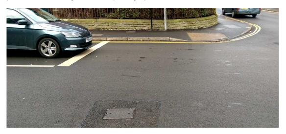
The ironwork cover is worn and polished, and there would be a likelihood of pedestrians slipping, falling and sustaining injury if stepping on the cover, particularly during or after inclement weather conditions.
